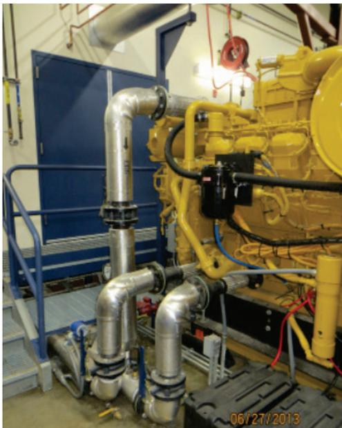
**Diesel engine with attached heat recovery system at the Point Lay Powerhouse in Alaska's North Slope Borough.**
