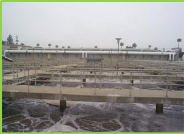
Hale Avenue Resource Recovery Facility (HARRF), City of Escondido
