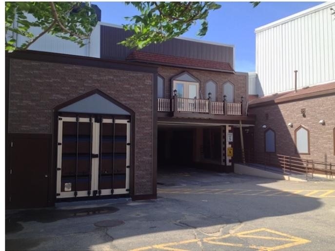
The CHP system is housed in a container that has been designed to fit the aesthetic design of nearby structures.
