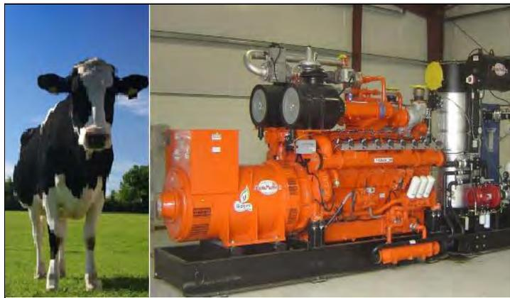
Manure can be transported to an anaerobic digester to produce biogas for use as fuel in a reciprocating engine to produce electrical energy and recoverable waste heat.
