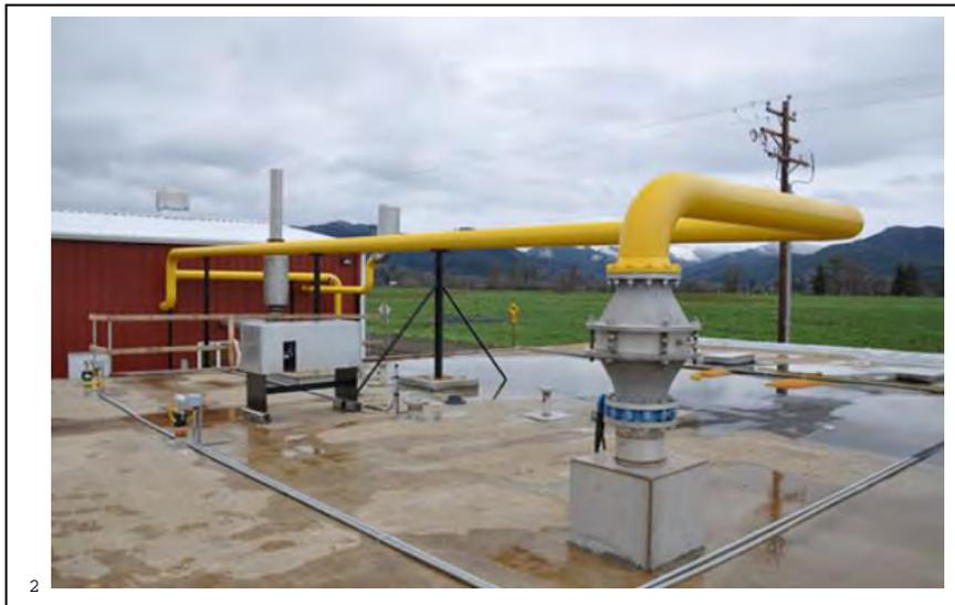
A methane transport pipeline conveys biogas to a 1,000 kW reciprocating engine at Farm Power-Tillamook
