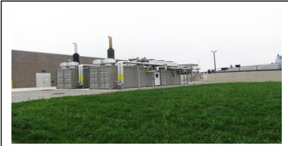
*Two 400kW Engine Driven CHP Systems with Heat Recovery
