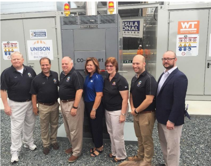
Governor Larry Hogan with Peninsula Regional Medical Center president and the MEA Team at 3.2 MW CHP plant
