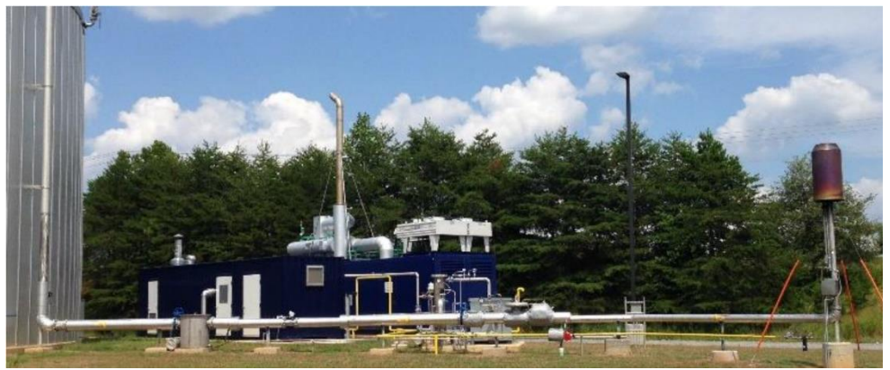
Anerobic Digester (far left), 400 kW Packaged CHP system (right side blue Module, Gas Flair (far right)
