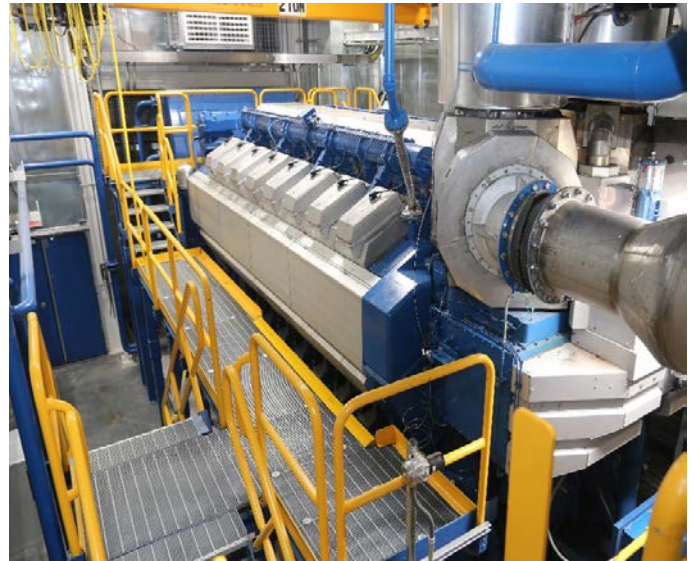
Wärtsilä 16-Cylinder Reciprocating Engine
