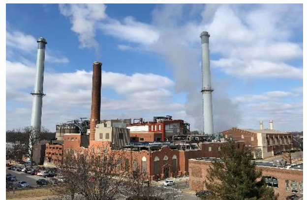
MU District Energy CHP Power Plant Photo Courtesy of University of Missouri
