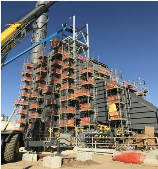
**Flint Hills recently constructed a state-of-the-art CHP system that uses natural gas and a heat recovery process to produce approximately 50 MW of electricity, or roughly 40% of the energy required to power the Pine Bend refinery. The facility is served under Xcel's revised standby service rider.**
